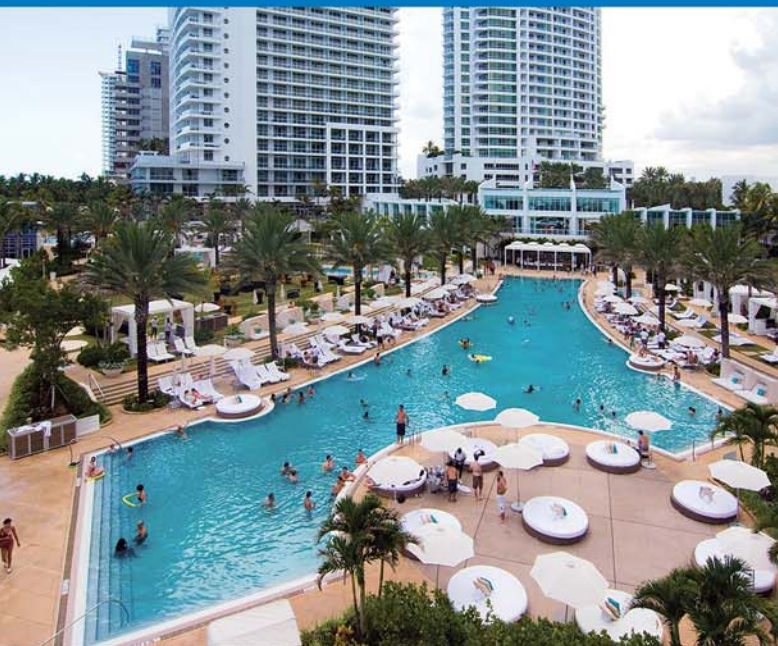
Above: Prestige guniting crews helped to create the magic of the fountains and pools at the recently renovated Fontainebleau in Miami.
