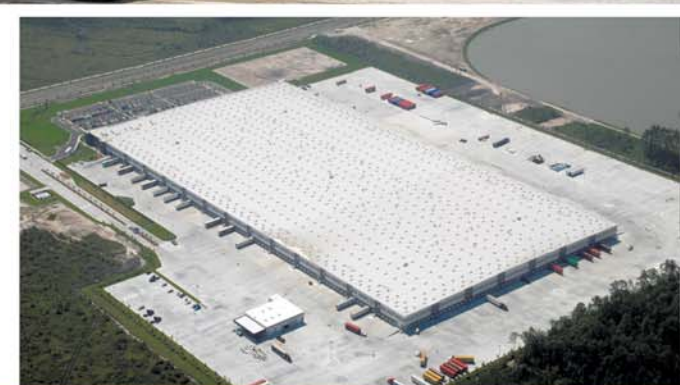
Right: Prestige concrete provided all the concrete for Bridgestone America's Tire Operations (BATO) one million square foot regional distribution center in Jacksonville.
