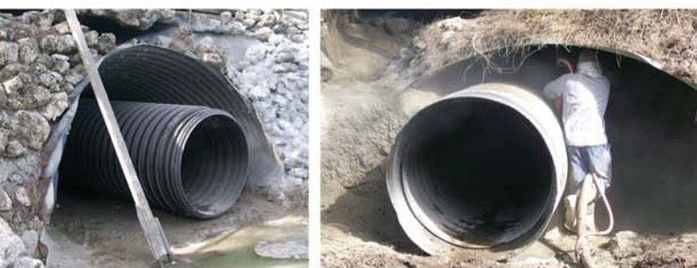
Below: Culvert Reconstruction, Ft. Meyers, FL.
